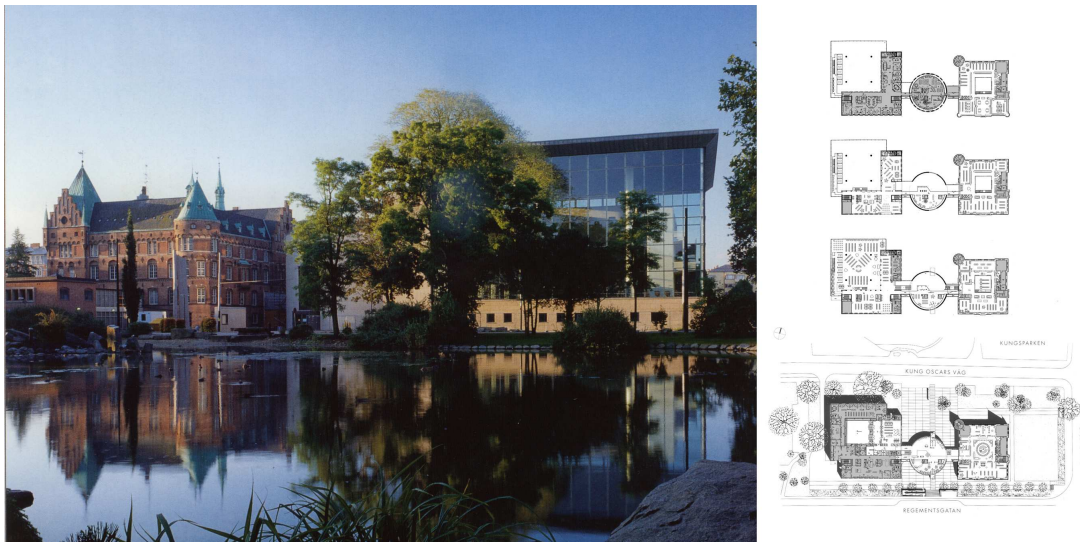
Figure - The City Library of Malmö - exterior photography and plans, presented in ascending order from the bottom up. Greyed areas are not accessible by the public.
